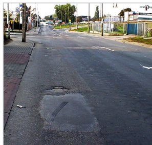
October 2006 — Initial road inspection. Visible damage on the wearing course, where even the pattern from the underlying hexagonal paving blocks can be seen.
