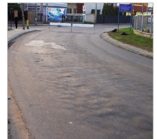
October 2006 — Initial road inspection. Visible damage on the wearing course, where even the pattern from the underlying hexagonal paving blocks can be seen.
