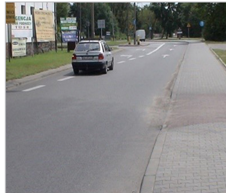
July 2007 — Inspection after eight months. Road remained in great condition.
