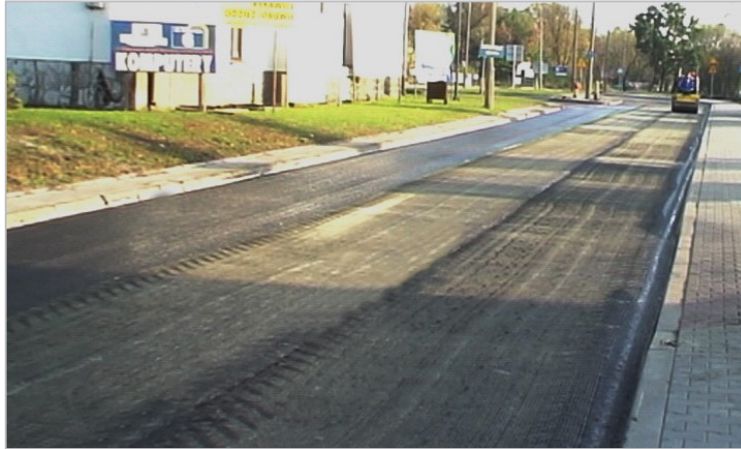
November 2006 — Carbophalt G asphalt reinforcement grid installation onto bitumen tack coat.
