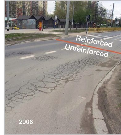
April 2008 — Inspection after 4.5 years. In the areas where Carbophalt G was installed, no damage was observed — in sharp contrast to sections of road with no grid.
