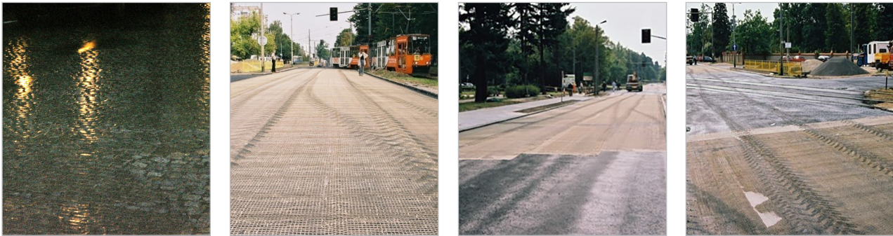
September 2003 — Simpson Strong-Tie asphalt reinforcement grid installation. The city of Wroclaw decided to repave the cobblestone road to ensure a more comfortable drive for road users.
