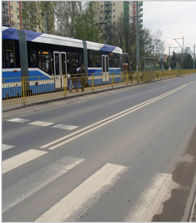
April 2008 — Inspection after 4.5 years. In the areas where Carbophalt G was installed, no damage was observed — in sharp contrast to sections of road with no grid.
