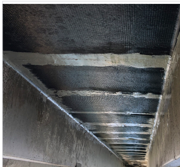
Completion of a reinforced and protected joint on the pier.
