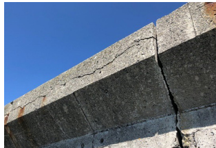
The cap of the seawall directs waves away from the buildings.
