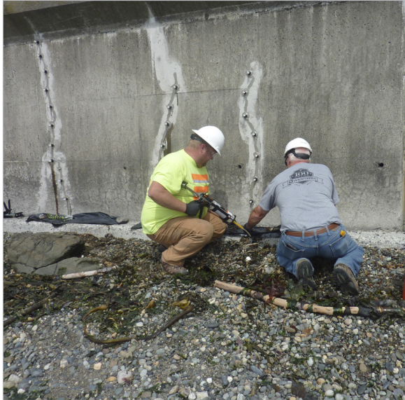
Major cracks were pressure-injected with structural epoxy.
