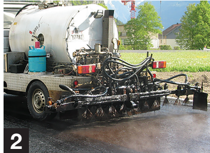
Application of the tack coat on the dry and dust-free surface.
