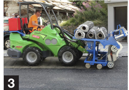
Grid application using the Simpson Strong-Tie grid installation machine.
