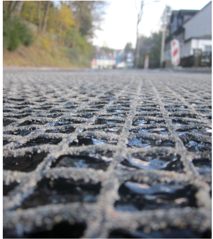
Grids are fully saturated with bitumen.
