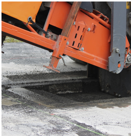
Milling the test area.
