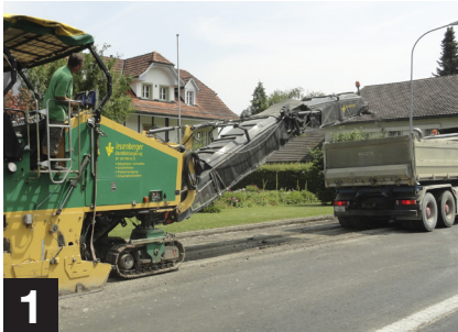
Surface preparation, such as milling.
