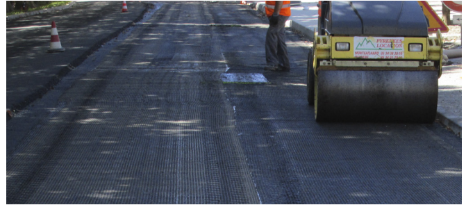
Complete surface application of Simpson Strong-Tie® reinforcement grid.
