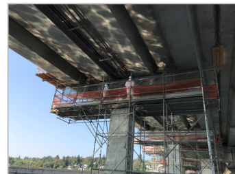
View of FRP girder reinforcement during installation.
