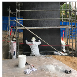
View of FRP column reinforcement during installation.
