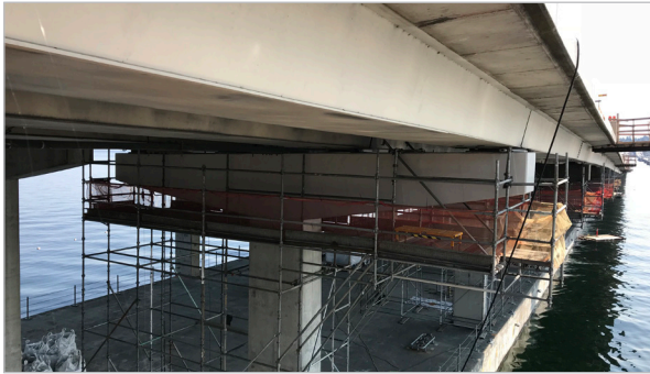
View of scaffolding around support bent in preparation for strengthening installations.
