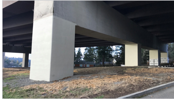
View of completed and coated FRP reinforcement at support columns.
