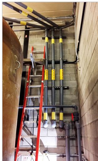
Wall obstructions prior to laminate installation.
