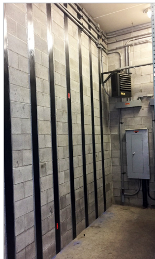
Installed laminate.
