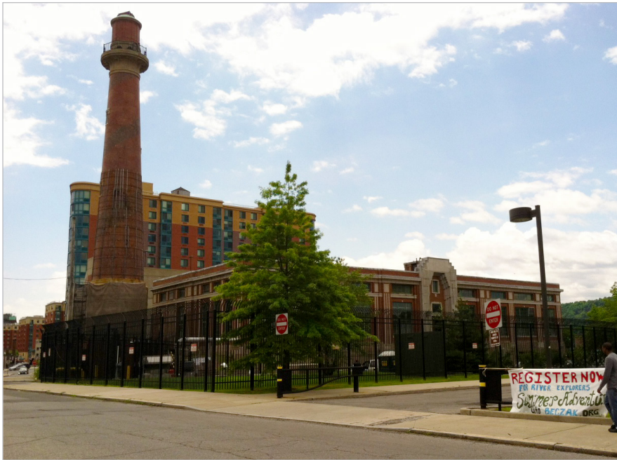
NYC mandates mitigation of flood hazards for wastewater infrastructure.
